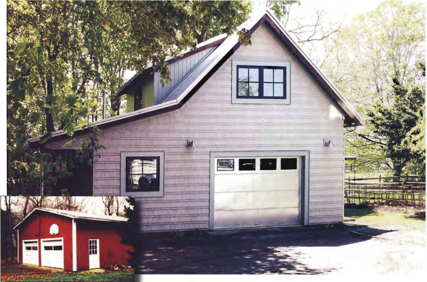
Before (inset) and after views of both the house and the faux barn garage (below), which became virtually a new building, with studio above and shop on the ground floor.
